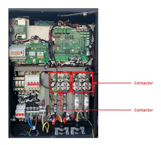
(2) Check pcb: There are small relays on the PCB that control the contactors. If they are damaged, it can also cause the fault, please try replacing the motherboard to solve the problem.
