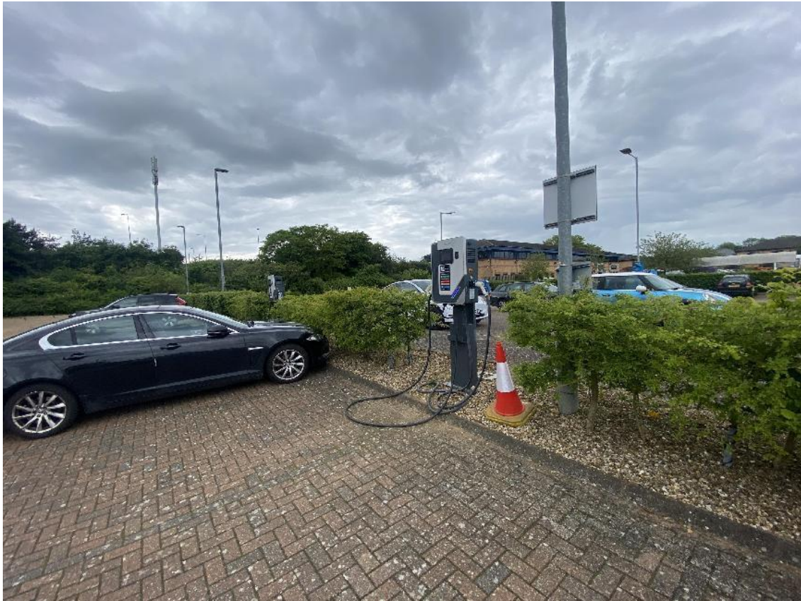
Two set of 40 kW ATESS EVD-40S/D DC EV chargers
