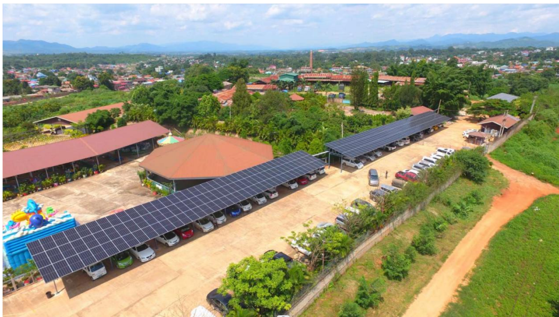
An ariel view of 121 kWp solar panels on the rooftop
