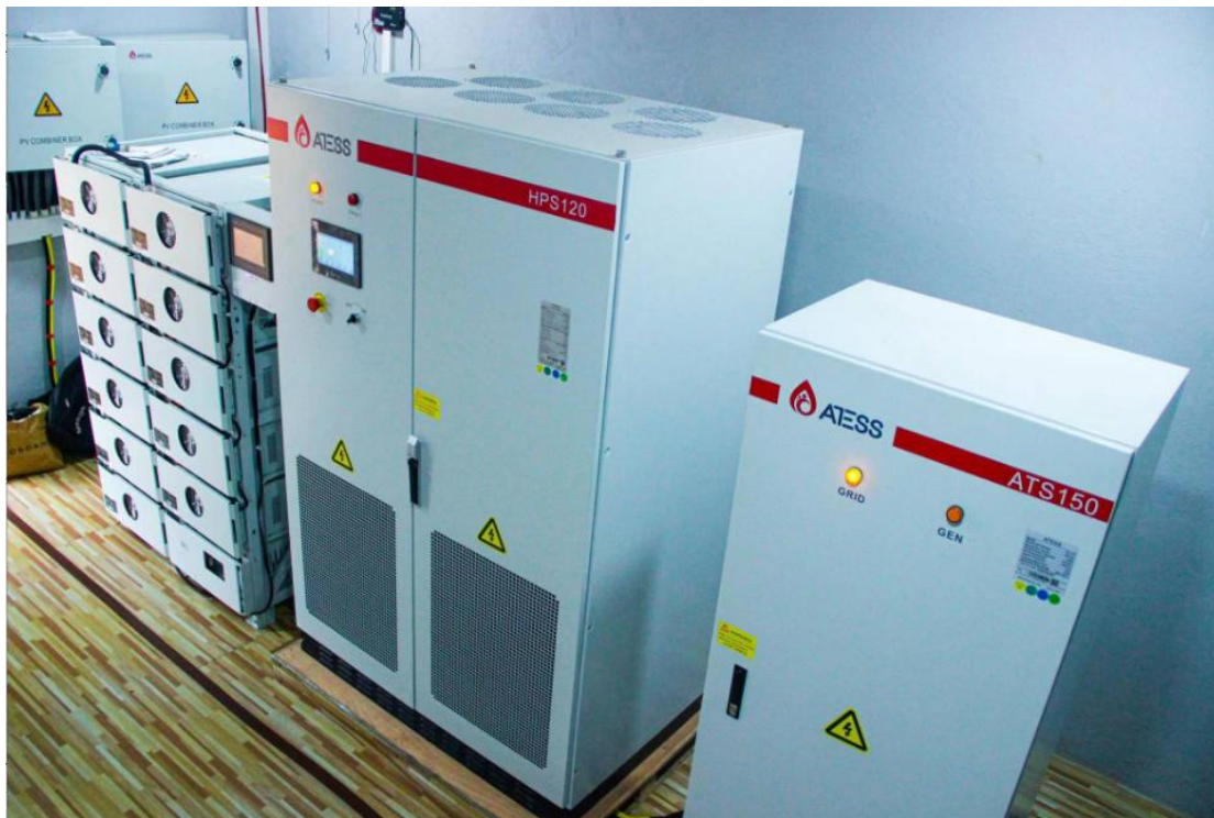
The 120 kW hybrid inverter on site
