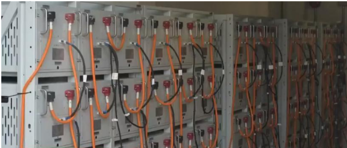
1,182.72 kWh ATESS battery system
