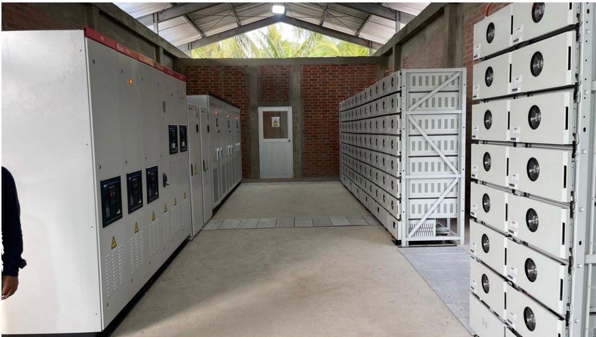
ATESS PCS + Bypass AC-Coupled BESS Solution
