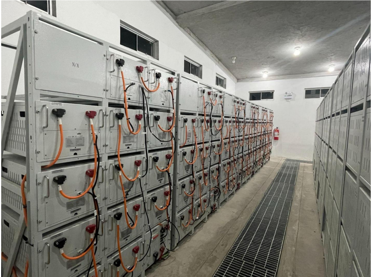
Total ATESS 16 sets of battery racks installed for the Bretaña project
