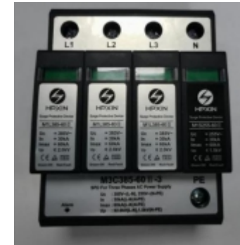
Fig: AC Surge protection device
